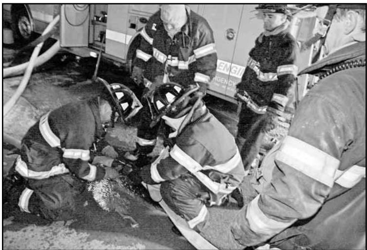
Reconfiguring hose from Engine 2 to feed Lodi 616 Foam Truck. Icy conditions made work difficult.
