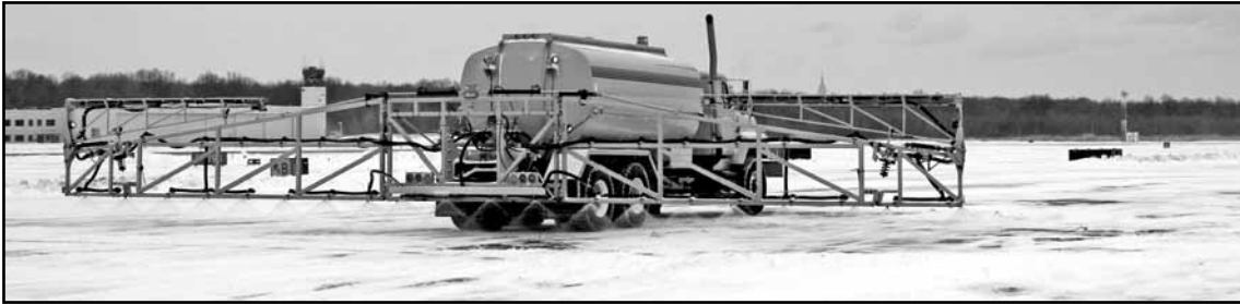
One 4,000 gallon truck sprays runways and has a boom that can open to 75', and a second 1,500 gallon truck sprays the taxiways. For this snow event, liquid potassium acetate was used. It is a protective coating for the runway and prevents ice and snow from bonding to the surface.
