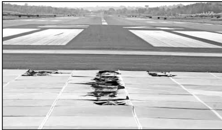
Damage done to the EMAS during the October 25th incident affected about 15 panels.
