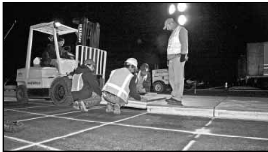
Installation of the arrestor bed began on the night of October 14th. The runway was closed and most of the work was done at night and during the weekends until completed.
