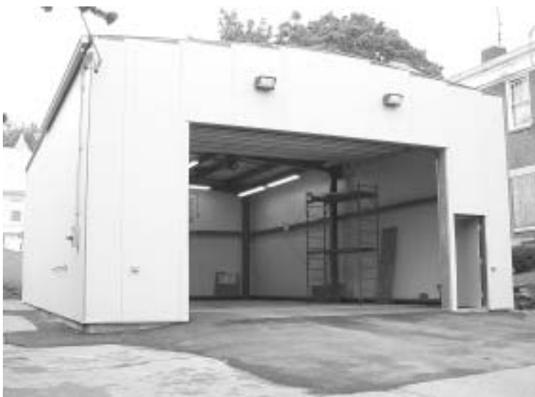
Construction of the larger Butler Building on Hamilton
