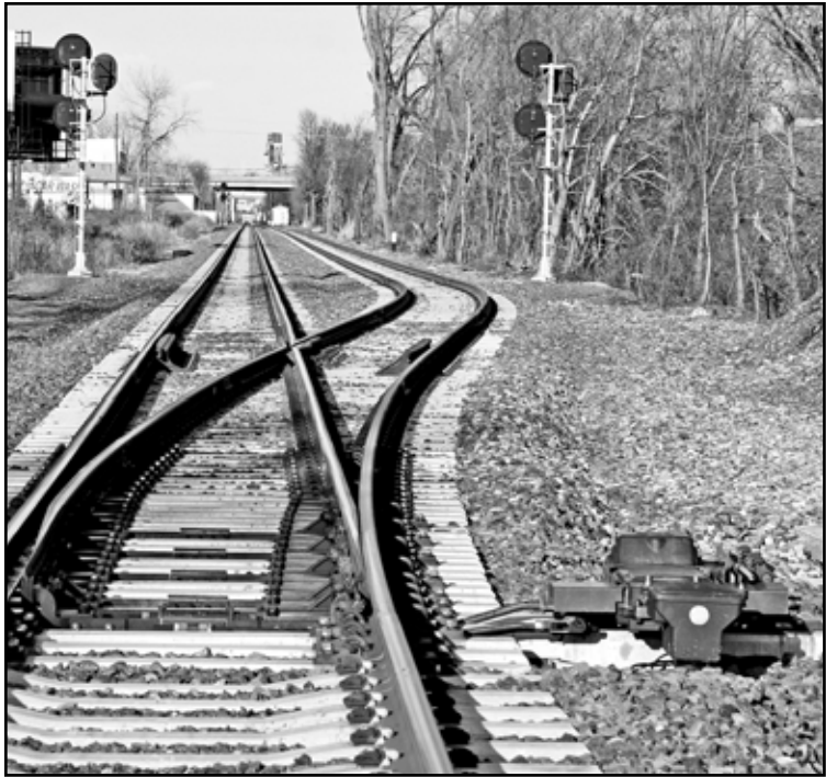
View of Hasbrouck Heights siding with new switch and signals, from Franklin Ave. towards Teterboro Station at Williams Ave.
