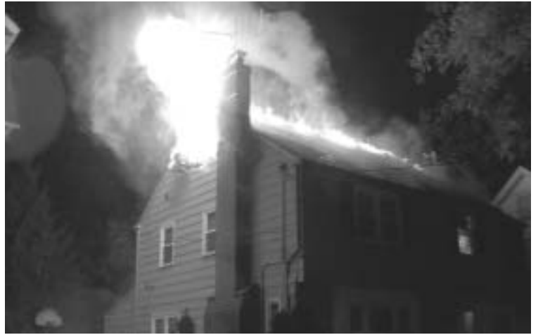
Working house fire on Madison Avenue November 4
