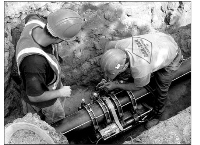
Replacing gas lines on Burton Avenue mid-August
