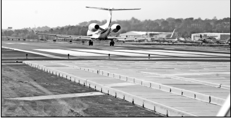
PA Installs Arrestor Beds at Teterboro -- December 2006 Issue
