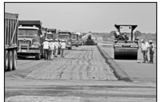
Teterboro's 6-24 Runway Gets Rehabilitated. November 2009
