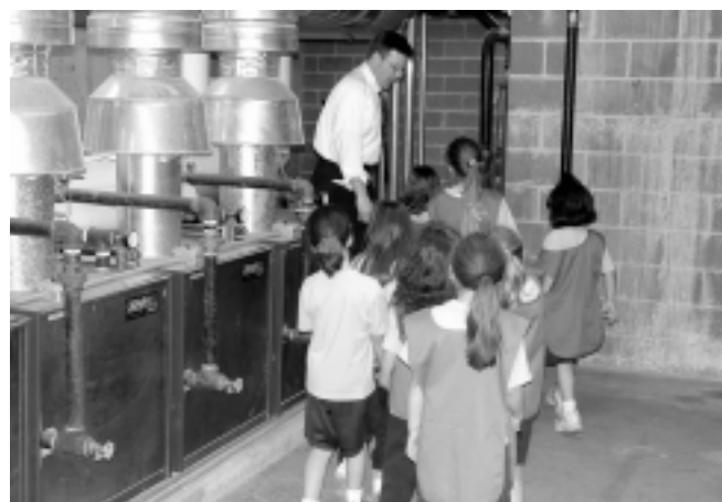
Mike showed the Daisies the utilities room.
