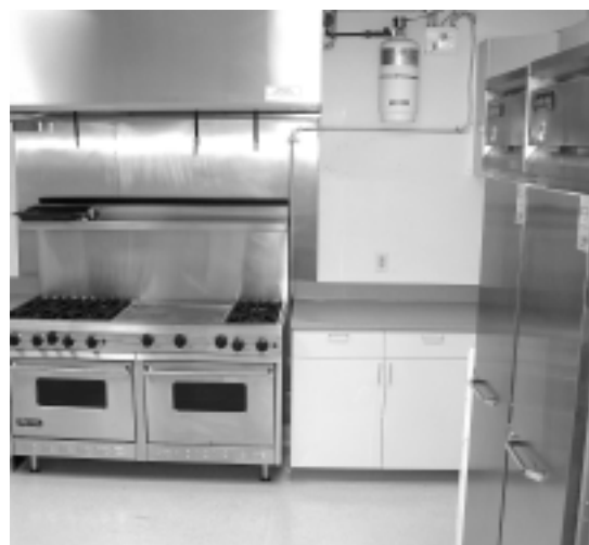
New kitchen facilities.
