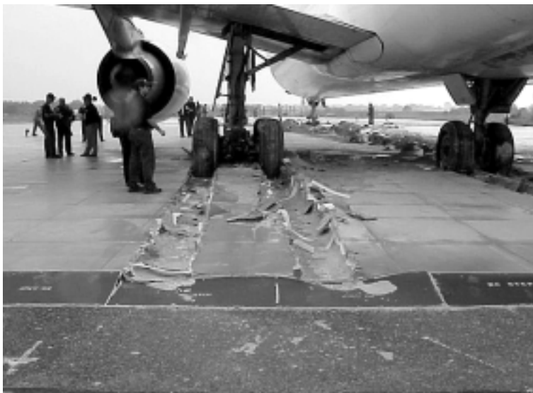
The Engineered Materials Arresting System at JFK successfully stopped this cargo plane on May 30, 2003. It also successfully stopped a commuter plane in 1999. Photo courtesy of the Port Authority of New York and New Jersey
