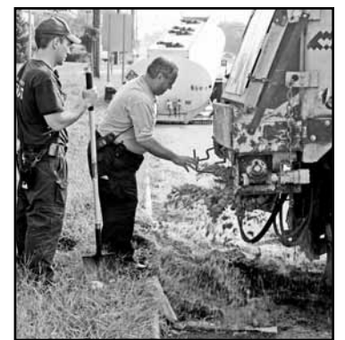
BC HAZ-MAT technicians and NJ DOT secure storm drain openings in case of spillage.
