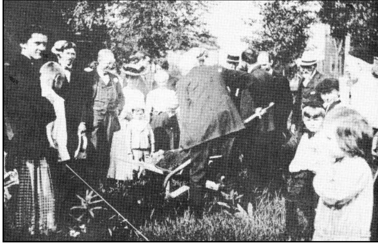
Ground Breaking for the new Church in June 1906. Every member took a turn at the shovel.
