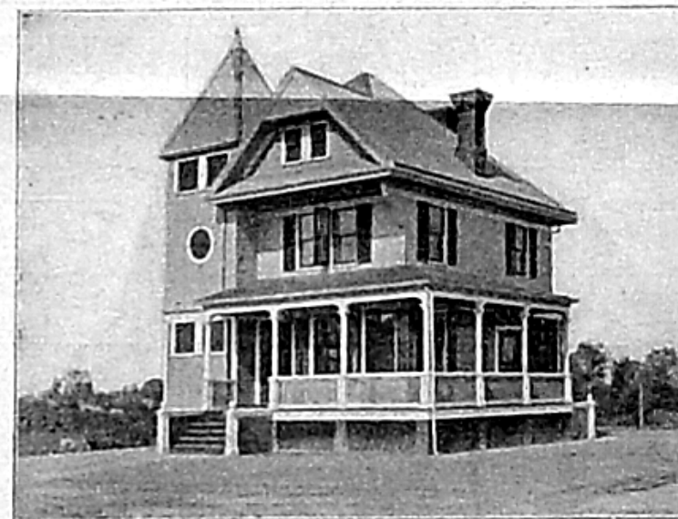
RESIDENCE OF DR. ELLSWORTH E. CONOVER, MADISON AVENUE.
